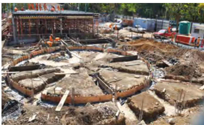
September: Construction begins in earnest
