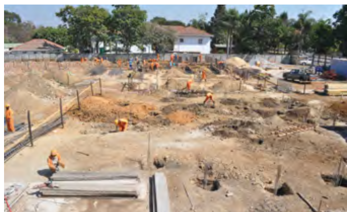
June: Laying the foundation pillars
