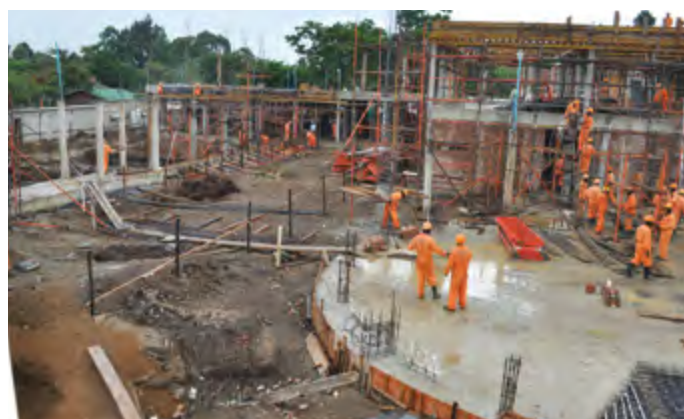
December: UP it goes!! The building rises
