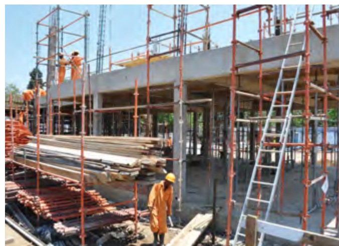
Construction work on the headquarters extension in progress
